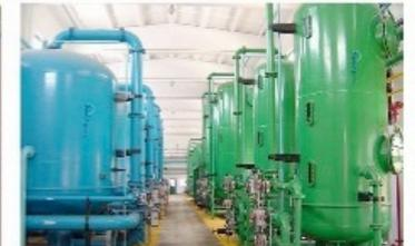
Ion exchange apparatus for chemical recapture of N and P from concentrated organic waste streams.
