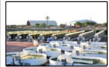
Large-scale algal culture facility for biological N and P recapture and bioenergy co-production from dilute waste streams at the Laboratory for Algae Research and Biotechnology, ASU Polytechnic.
